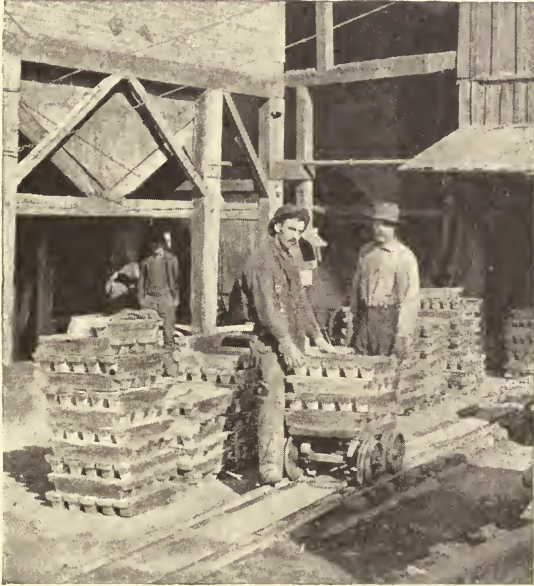
BULLION AT THE AMERICAN SMELTER, LEADVILLE, COLORADO
